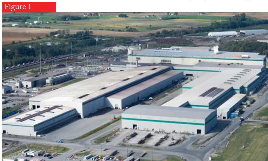
Overview of SDI Facility
