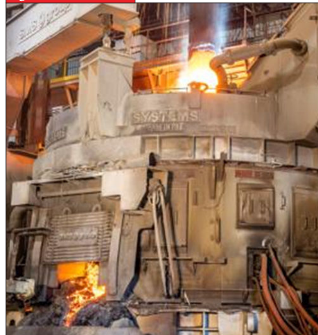
Systems Spray-Cooled Upper Shell (Sidewall) and Roof in Operation
